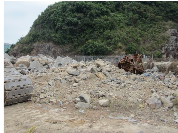
Photo 4 - Tarpaulin sheets to cover open stockpiles to prevent dust generation were absent from the construction site.
