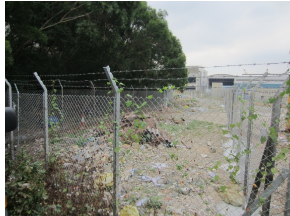
Photo 2 - Fences were erected along both sides of the land duct alignment
